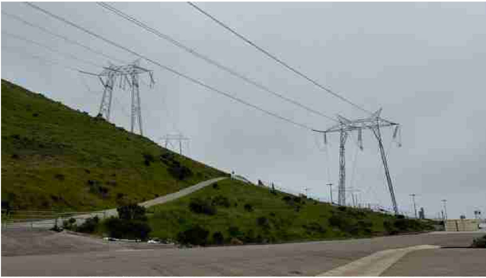
High-voltage lines carry electricity from Diablo Canyon nuclear power plant to a switchyard and then out to California's energy grid.
