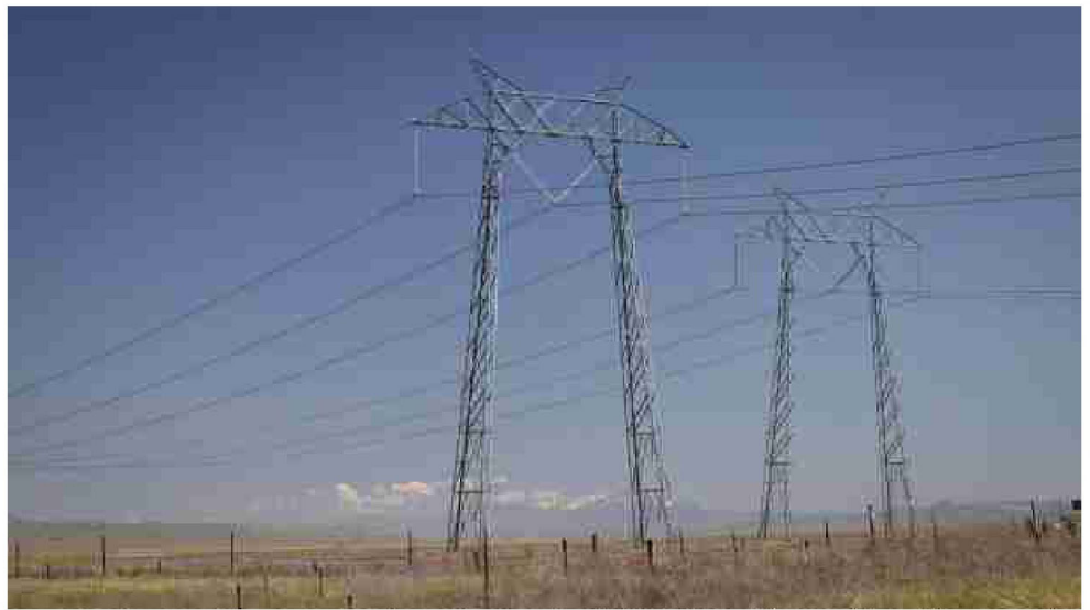
Power lines from Diablo Canyon nuclear power plant cross Soda Lake with Mt. Pinos covered in snow in the distance on April 3, 2024, as wildflowers bloom on the Carrizo Plain.
